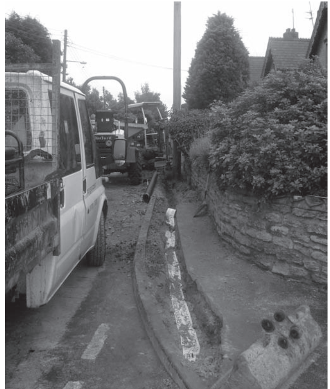
Trenches being dug for the underground low voltage cables which are to replace the existing overhead cables in Main Street, South Rauceby.
